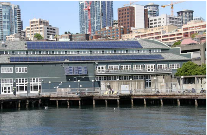
247-solar panel array installed on the roof of Pier 59 in 2013.
